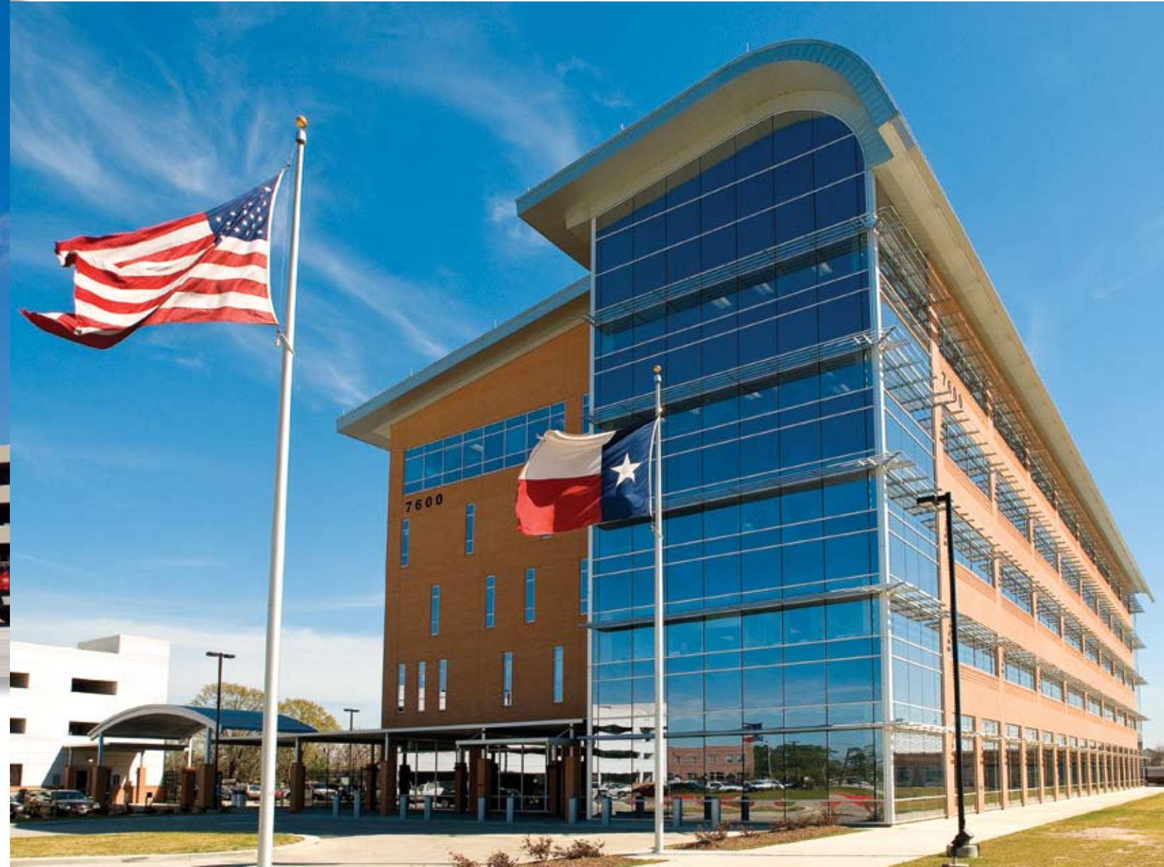
PROJECT: Texas Department of Transportation - Houston Headquarters ARCHITECT: Gensler CONTRACTOR: Gilbane Building Company OWNER: Texas Department of Transportation SCOPE: Curtain Wall, Window Walls, Aluminum Sunshades
