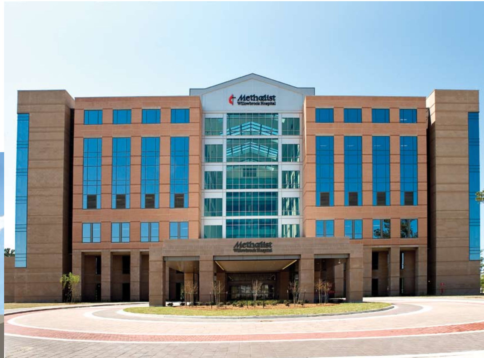
PROJECT: Methodist Willowbrook Hospital Expansion ARCHITECT: Hellmuth Obata Kassabaum, Inc. CONTRACTOR: Vaughn Construction Company OWNER: The Methodist Hospital SCOPE: Curtain Wall, AGC Aluminum Composite Panel System, Custom Interior Art Glass, Glass with Integral Blinds.
