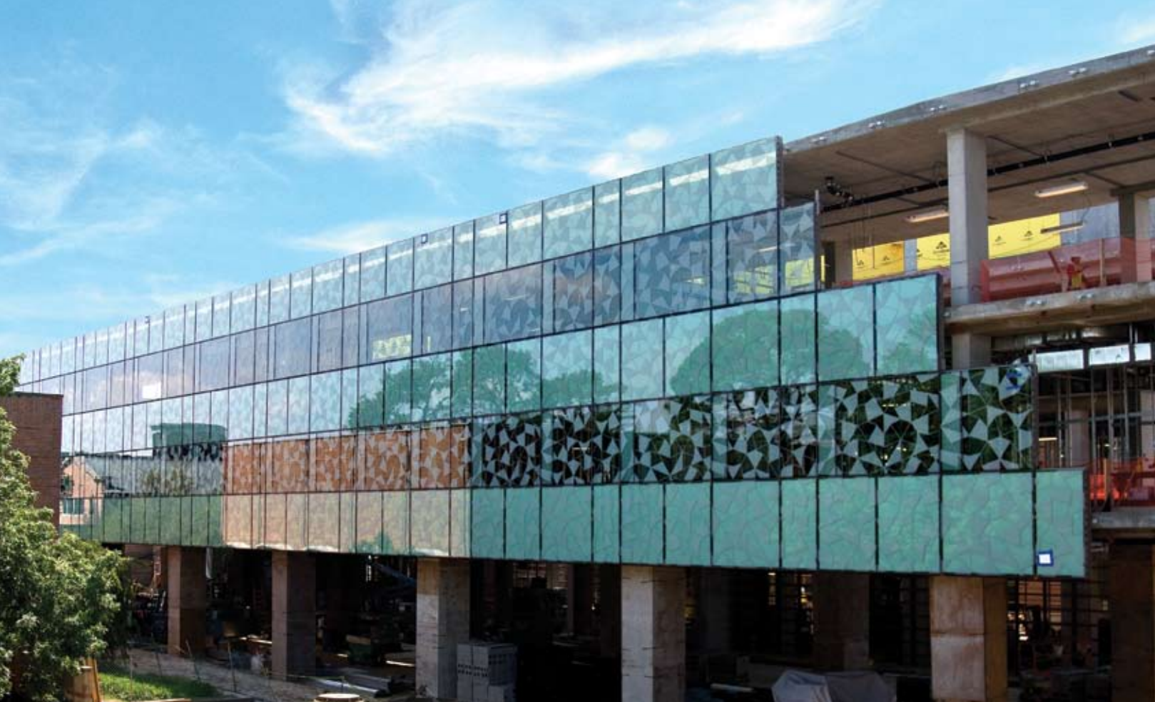
PROJECT: Rice University Brockman Hall for Physics (In Progress) ARCHITECT: Kieran Timberlake Associates LLC CONTRACTOR: Gilbane Building Company OWNER: Rice University SCOPE: AGC Custom Unitized Curtain Wall, AGC Aluminum Composite Panels, AGC Custom Sunshades, Terracotta Clay Baguettes, Suspended Glass Ceiling.
