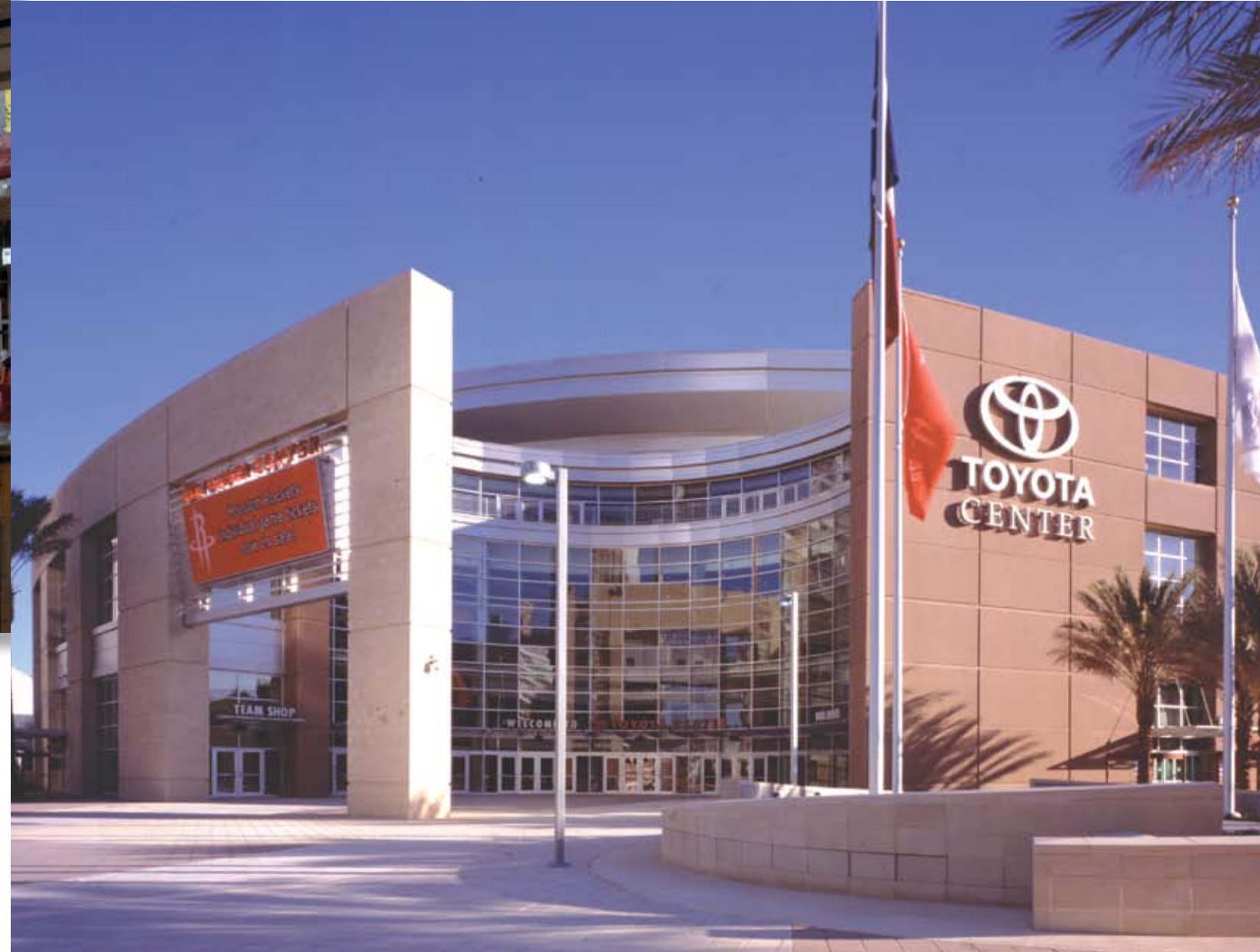
PROJECT: Toyota Center ARCHITECT: Hellmuth, Obata + Kassabaum, L.P./Morris Architects CONTRACTOR: Hunt Construction Group OWNER: Houston Sports Authority SCOPE: Curtain Wall, Window Wall
