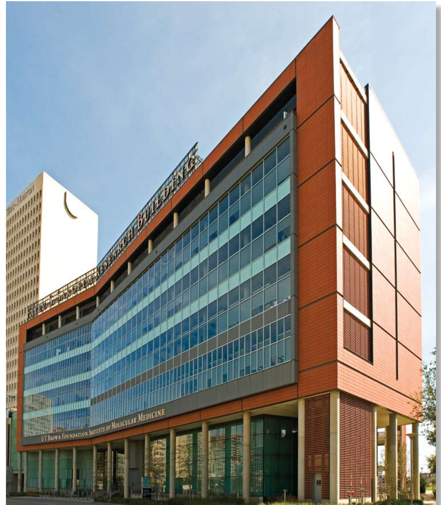
PROJECT: University of Texas Institute of Molecular Medicine ARCHITECT: Berkebile Nelson Immenschuh McDowell CONTRACTOR: Vaughn Construction Company OWNER: University of Texas Health Science SCOPE: Curtain Wall, Window Wall, Terracotta Tile, Aluminum Sunshades
