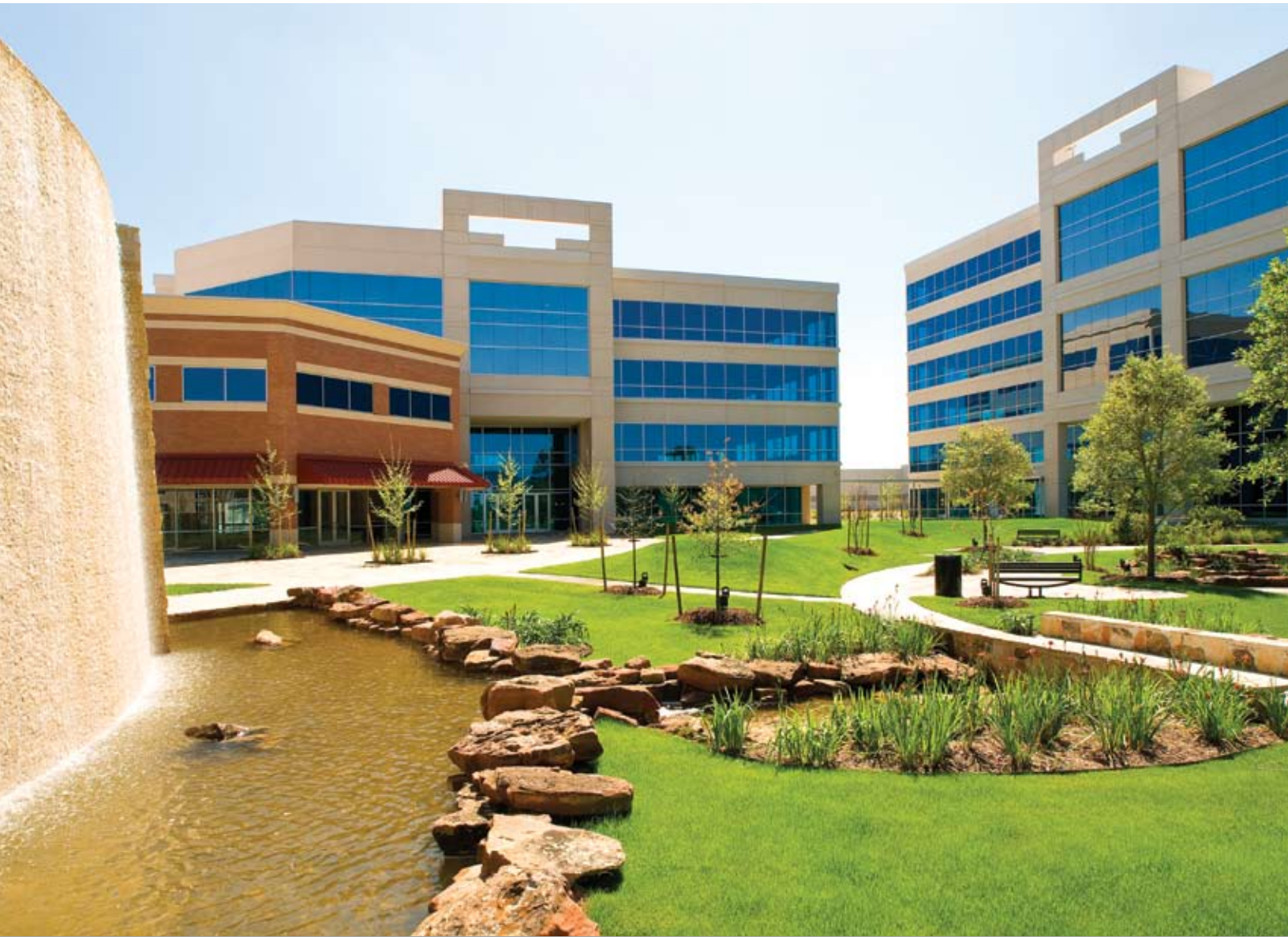
PROJECT: Remington Square ARCHITECT: Consolidated Architecture & Planning Services, Inc. CONTRACTOR: E.E. Reed Construction, LP OWNER: Sun Life Assurance Company of Canada SCOPE: Curtain Wall, Window Wall
