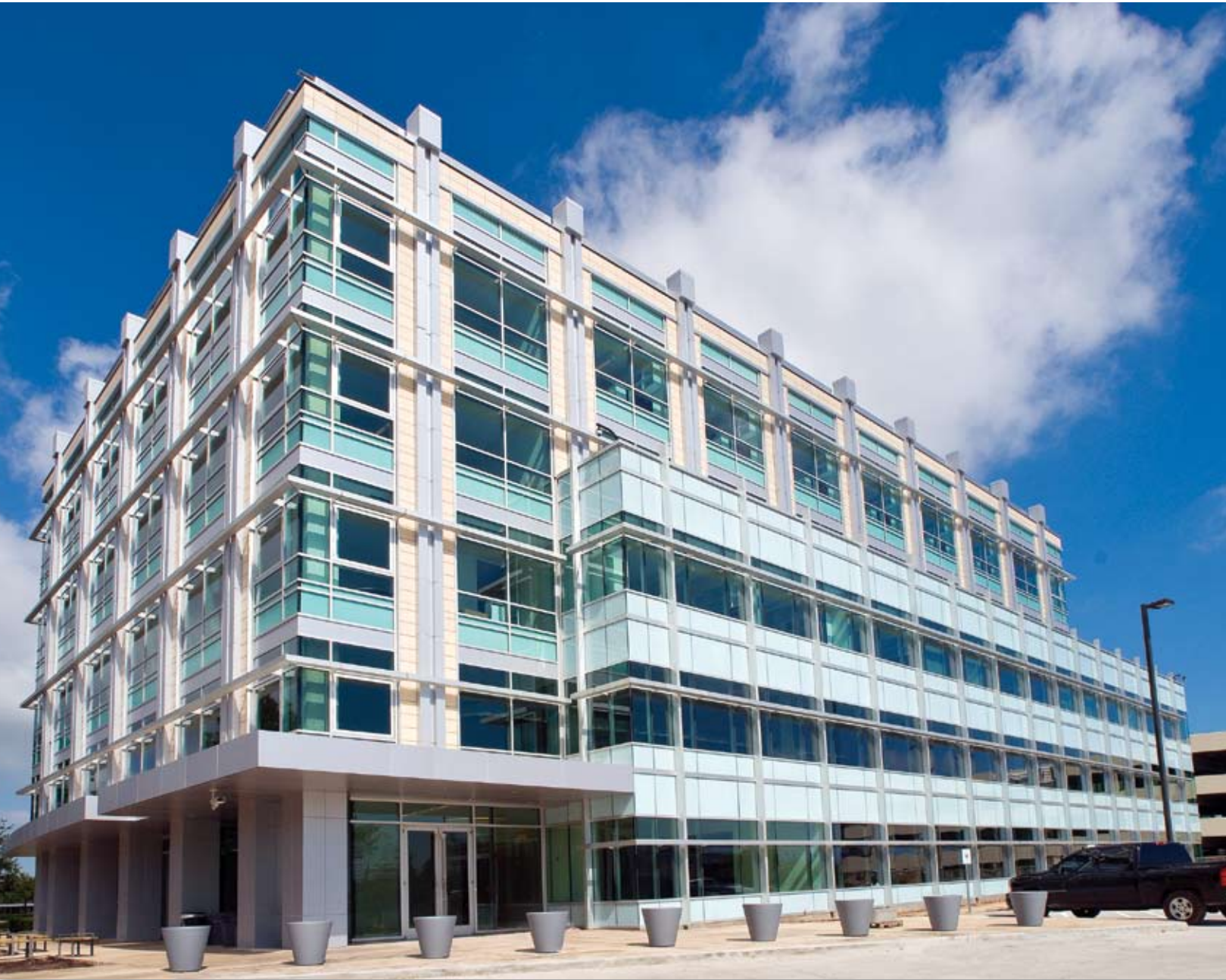
PROJECT: Seismic Exchange Phase 3 ARCHITECT: Powers Brown Architects CONTRACTOR: Rosenberger Construction OWNER: Boulder Management, LTD SCOPE: Curtain Wall, Terracotta Tile, Aluminum Sunshades, AGC Aluminum Panels
