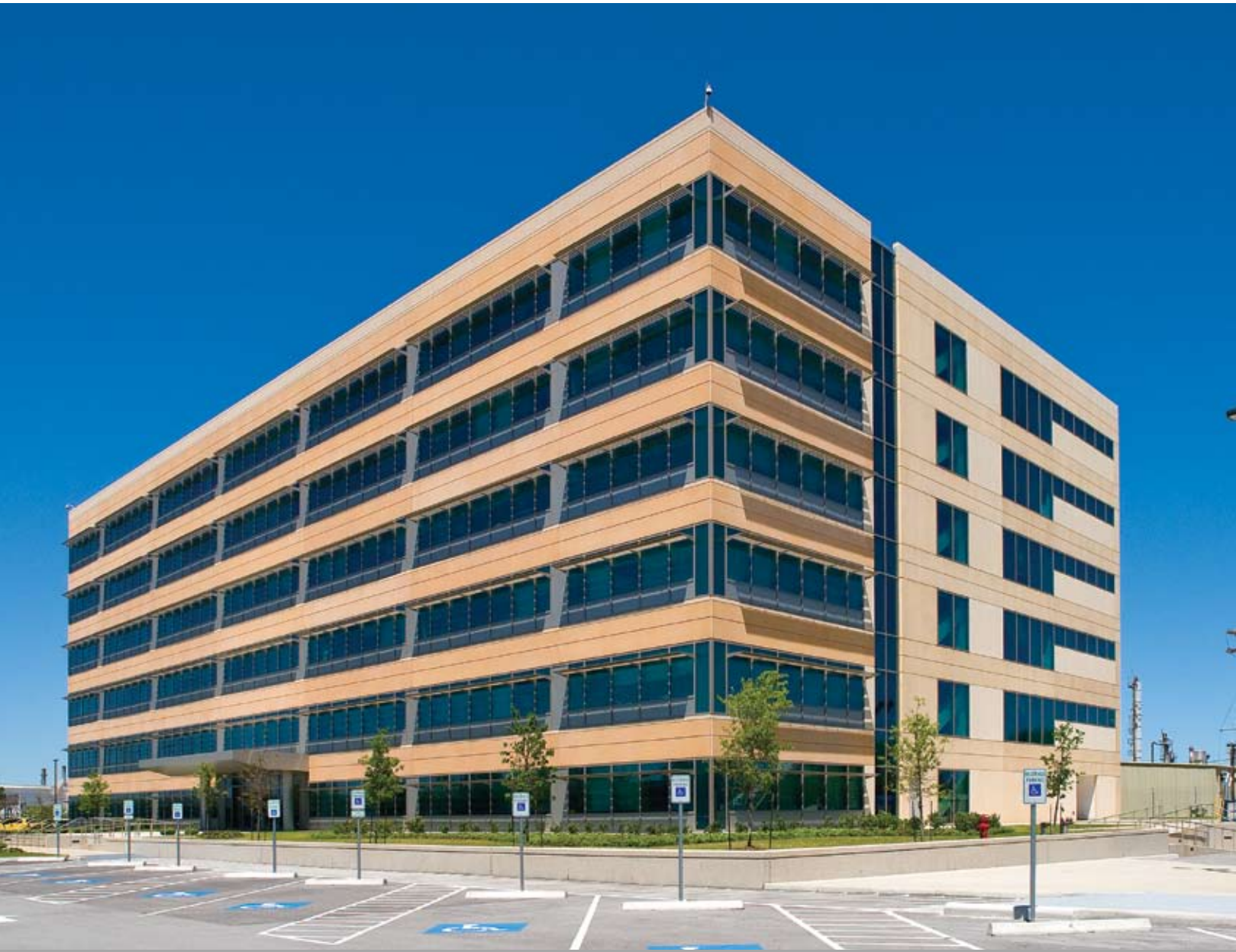
PROJECT: Shell Deer Park ARCHITECT: Gensler CONTRACTOR: J.E. Dunn of Texas, Inc. OWNER: Shell Global Solutions, Inc. SCOPE: AGC Custom Blast Resistant Curtain Wall, AGC Custom Blast Resistant Window Wall, AGC Aluminum Sunshades
