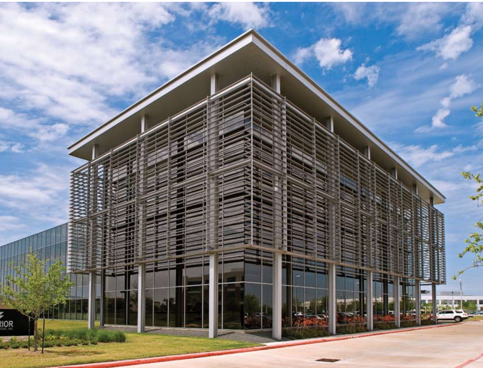
PROJECT: Westway Park Office Building ARCHITECT: Kirksey Architecture CONTRACTOR: Satterfield & Pontikes Construction, Inc. OWNER: Satterfield & Pontikes Construction, Inc. SCOPE: Curtain Wall, Window Wall, AGC Aluminum Sunshades
