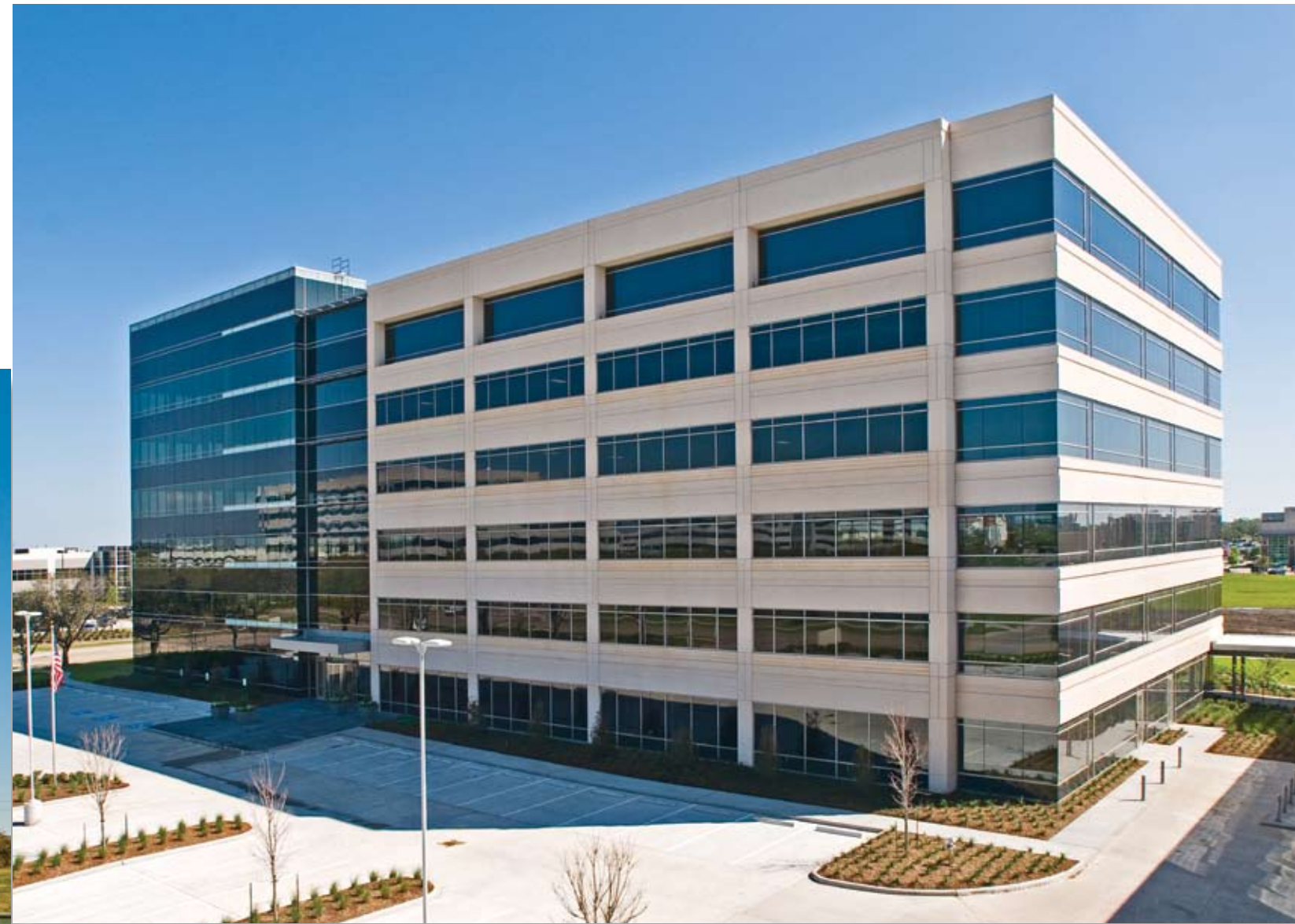
PROJECT: One Oak Park ARCHITECT: Gensler CONTRACTOR: Tribble & Stephens Constructors, LTD. OWNER: CRP/MK Oak Park LLC SCOPE: Curtain Wall, Window Wall, Aluminum Sunshades
