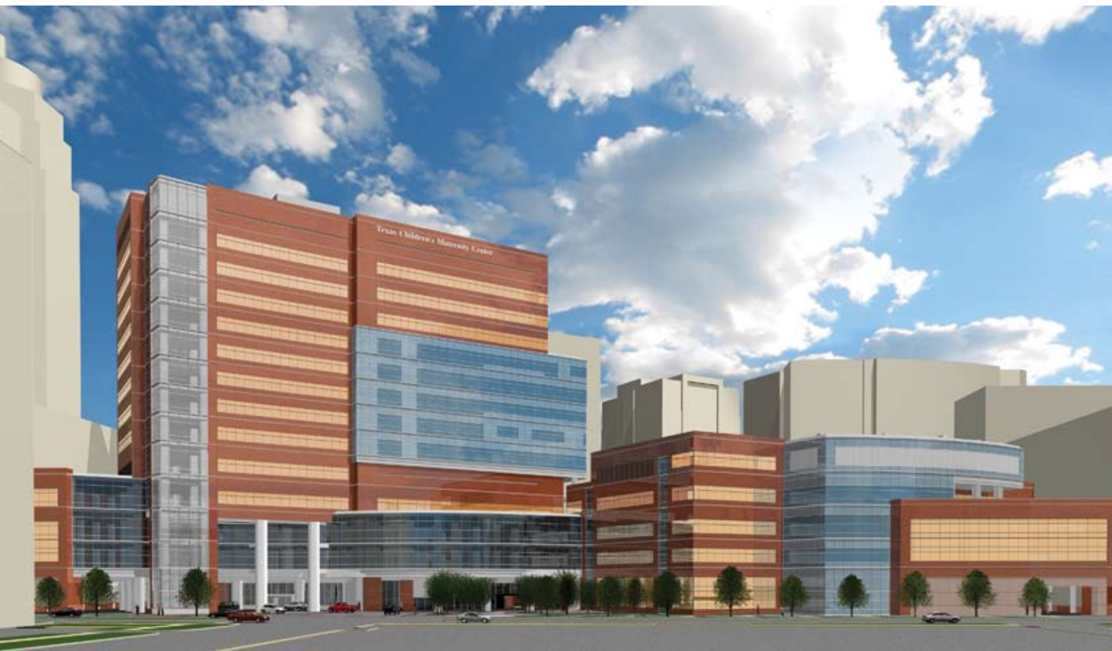
PROJECT: Texas Children's Hospital Maternity Center ARCHITECT: FKP Architects CONTRACTOR: W.S. Bellows Construction Corporation OWNER: Texas Children's Hospital SCOPE: AGC Custom Designed Unitized Curtain Wall, AGC Custom Designed Unitized Ribbon Window System, Aluminum Stick System, Aluminum AGC Aluminum Plate Panels.
