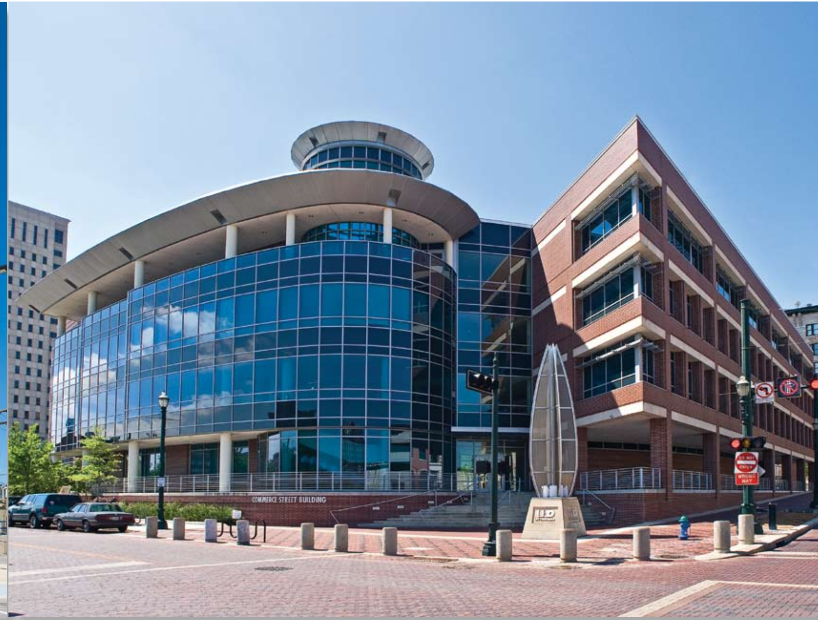
PROJECT: U of H Downtown New Classroom Bldg ARCHITECT: Gensler CONTRACTOR: Spaw Glass OWNER: University of Houston SCOPE: Curtain Wall, Window Wall, Aluminum Sunshades
